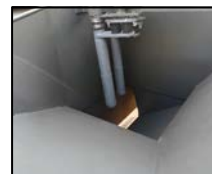
Needle Vibrators in Mould Box
